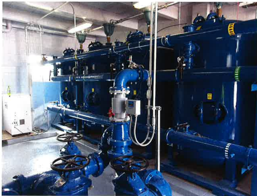
Photo 3: New iron filter in Well #2, part of 2017 upgrade
