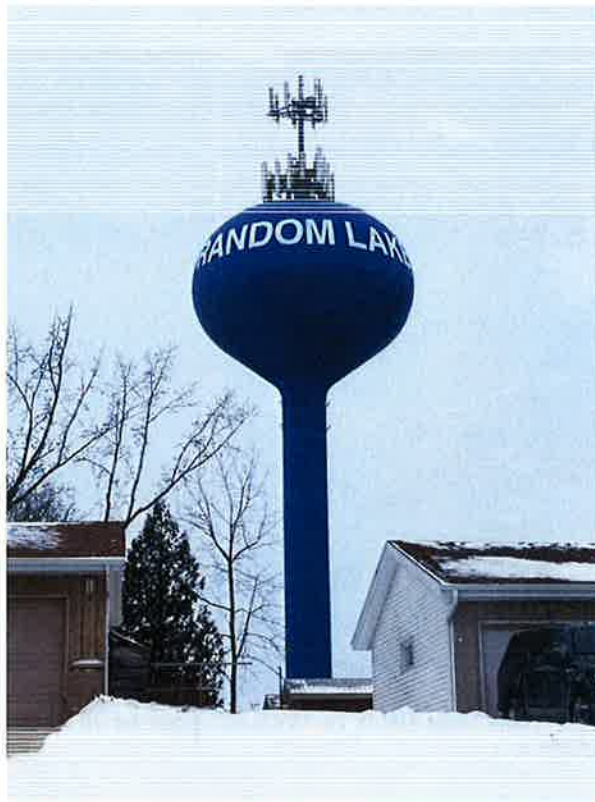
Photo 4: Elevated storage tank in Random Lake
